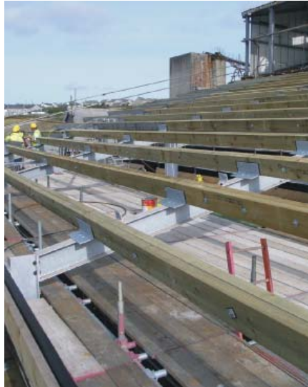
With new timbers in place the roof starts to take shape
