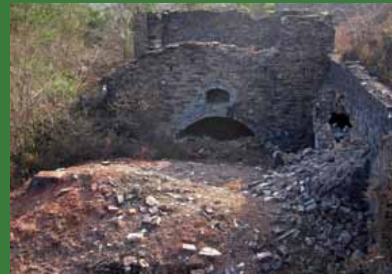
Above - A mound of earth and rubble in front of a Brunton arsenic calciner conceals the arsenic refiner before the start of building conservation works (Colin Buck © Cornwall Council)
