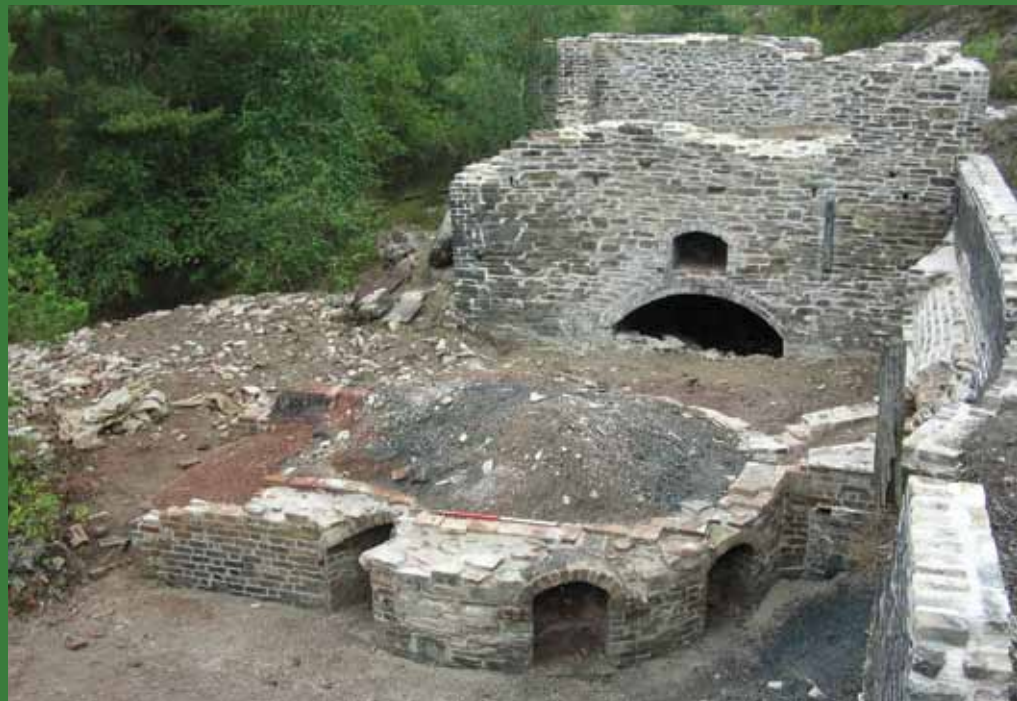
Above - A mound of earth and rubble in front of a Brunton arsenic calciner conceals the arsenic refiner before the start of building conservation works (Colin Buck © Cornwall Council)
