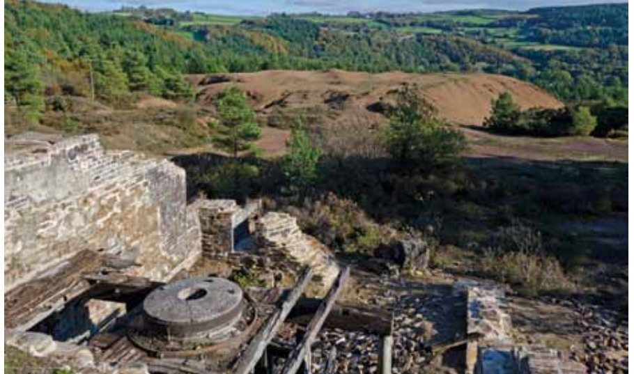
Above - The remains of the rare arsenic grinder at Devon Great Consols, now conserved, with the extensive mine processing waste dumps beyond
