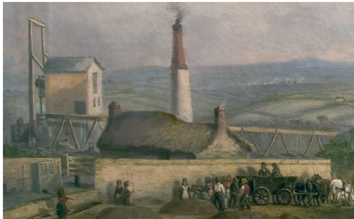
This detailed view shows an elevated timber launder (centre left and right) carrying water from the engine shaft where it has just been pumped; the artist must have observed that such launders often leaked and has incorporated this into the composition
