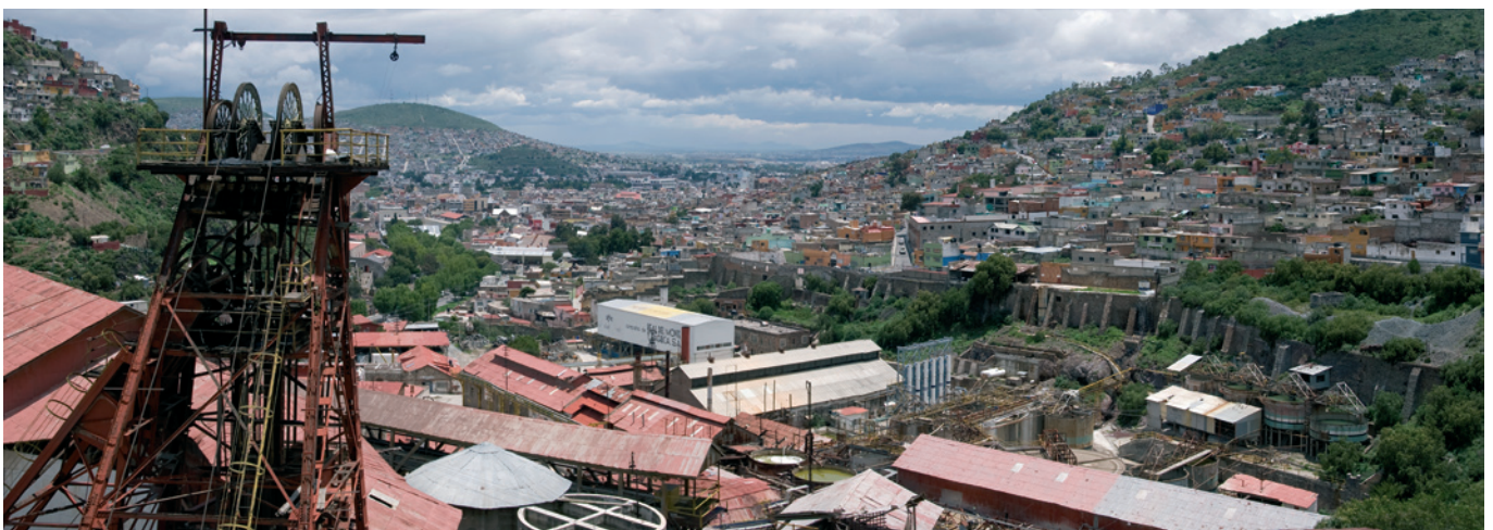
The Loreto Mine and mill complex overlooking Pachuca de Soto; this was the last major ore processing mill to operate in the area. Nearby is the location where the patio silver amalgamation process is reputed to have first been introduced into Latin America (c.1557). For this, argentiferous ores were mixed with mercury to achieve the required separation of the valuable silver. This method remained in use until the introduction of the cyanide process at the beginning of the twentieth century when the US Smelting Refining and Mining Company acquired the Cia. de Real del Monte y Pachuca
