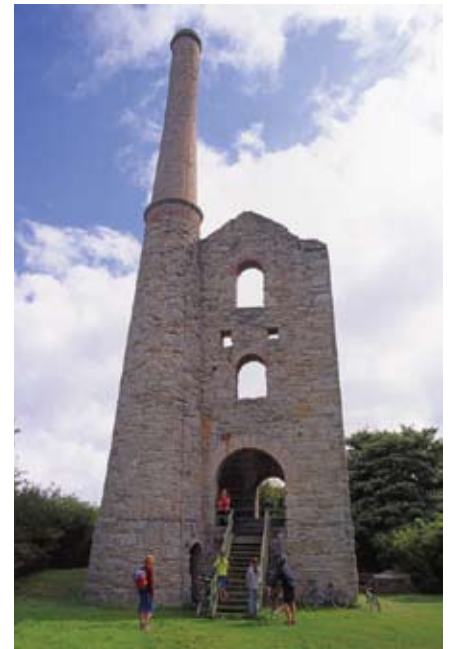
Hawke's Shaft engine house, Killifreth Mine near Chacewater (Paul Watts © Cornwall Council)
