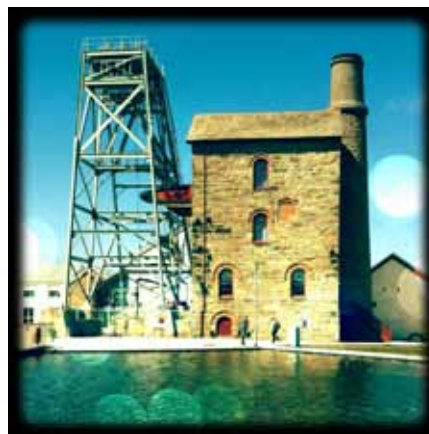
The Robinson's Shaft pumping engine, the last to have worked on a metal mine in Cornwall © Matt Silver
