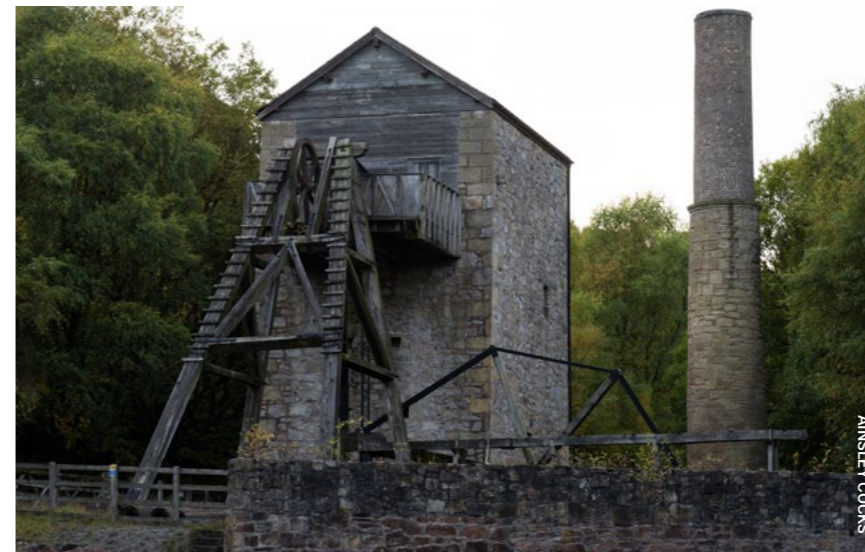
The preserved Cornish-type pumping engine house at Minera Mines, Wrexham, Wales. A tangible reminder of Cornish involvement at mines across Britain in the nineteenth century
