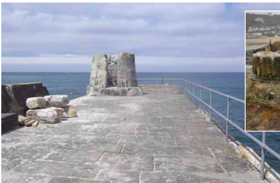
Above and left: the northern extent of the Western Breakwater featuring the Forward Observation Hut, which is being rebuilt using the original granite; inset image shows the extent of the damage caused in January (A. Brigden)
