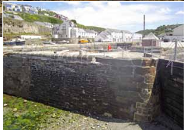
Above: the 'wave breaker' inside the Harbour following the reinstatement of the cast concrete coping sections, most of which had been displaced (A. Brigden). Note the date '1946' on the cement coping to the right
