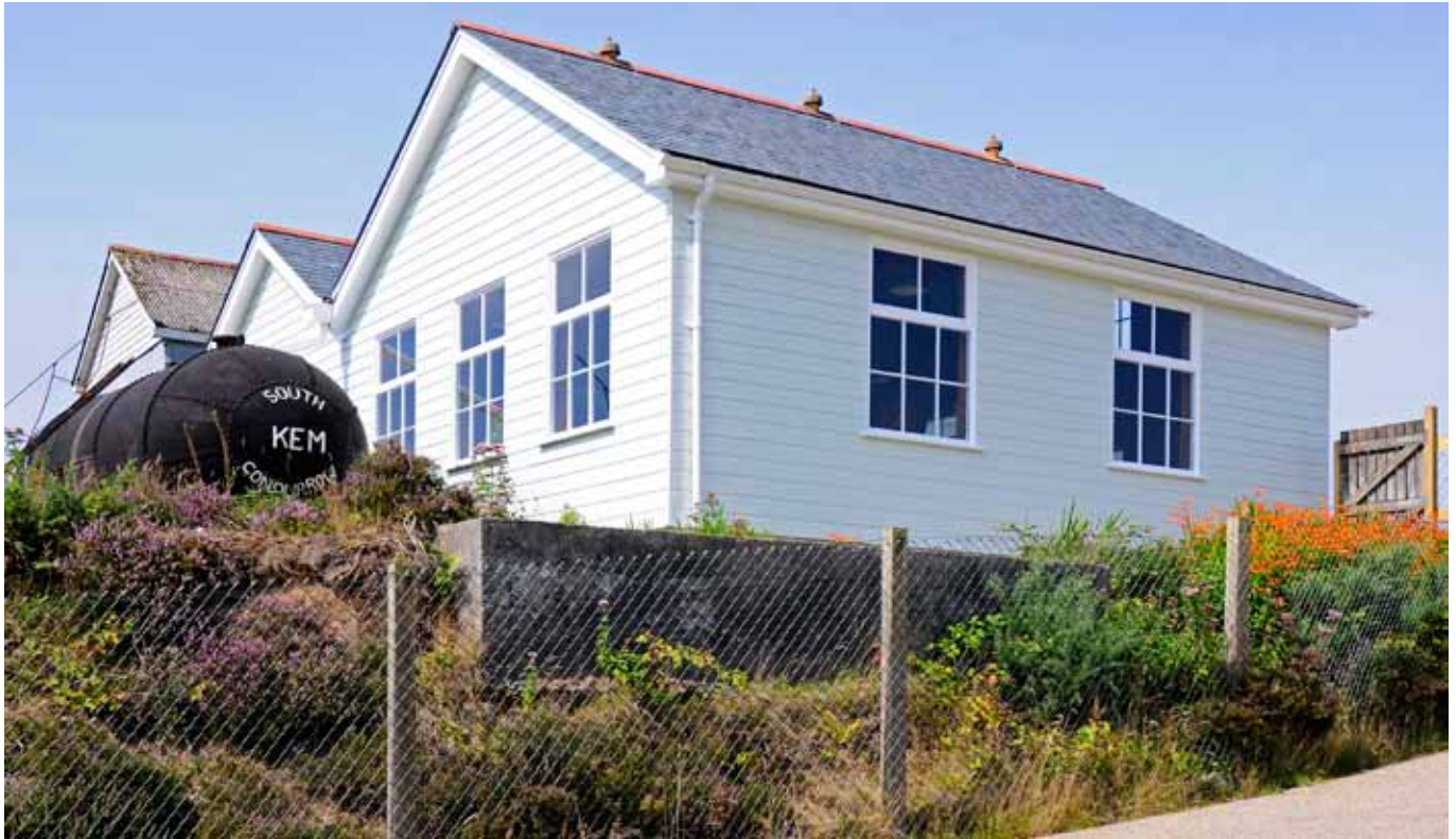
Winder and Compressor houses build in 2010 as part of the World Heritage Site 'Discover the Extraordinary' project
