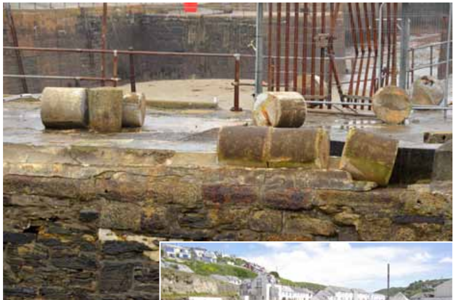
Above: the 'wave breaker' inside the Harbour following the reinstatement of the cast concrete coping sections, most of which had been displaced (A. Brigden). Note the date '1946' on the cement coping to the right
