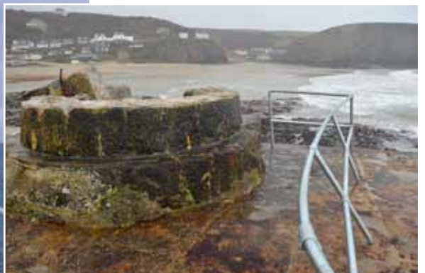
Above and left: the northern extent of the Western Breakwater featuring the Forward Observation Hut, which is being rebuilt using the original granite; inset image shows the extent of the damage caused in January (A. Brigden)
