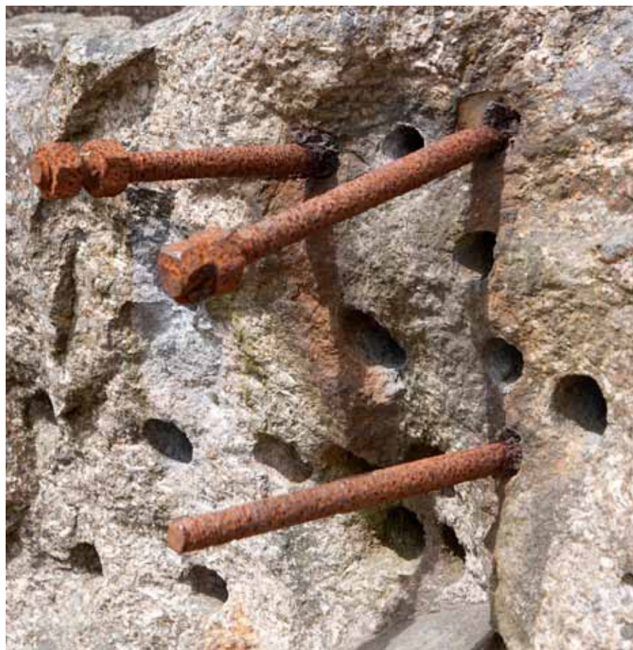
Above: Granite block – probably used to train students in the skill of compressed air machine drilling Top: The weather-boarded Carpenters' Shop and Machine Room, adjoining (Images: Steve Hartgroves, Ainsley Cocks, Convergence Cornwall)
