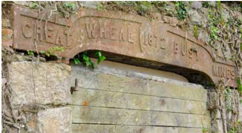
One of the two impressive cast iron lintels above entrances to the Smithy, anticipating good fortune for the mine in 1872 which unfortunately did not materialise; the mine was to close again by the end of July the following year
