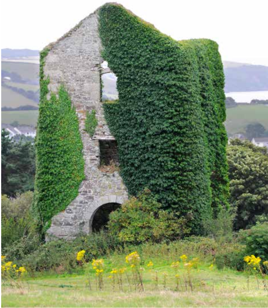
A closer view of Austen's 80 inch cylinder engine house at Fowey Consols
