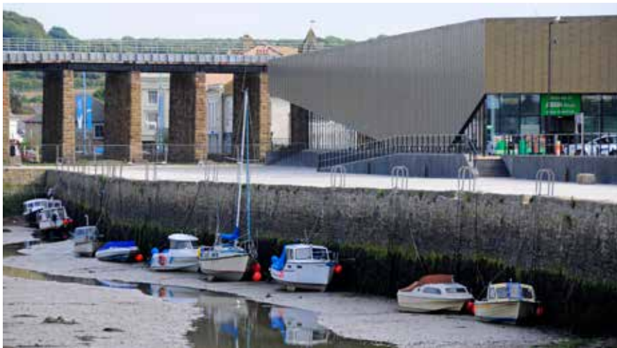
Following completion of the store and extensive wall repair
