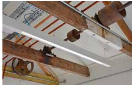
Two views of the completed workspace units within the weather-boarded Carpenters' Shop and Machine Room; original features such as the overhead line-shafting here – formerly providing machine power – have been retained
