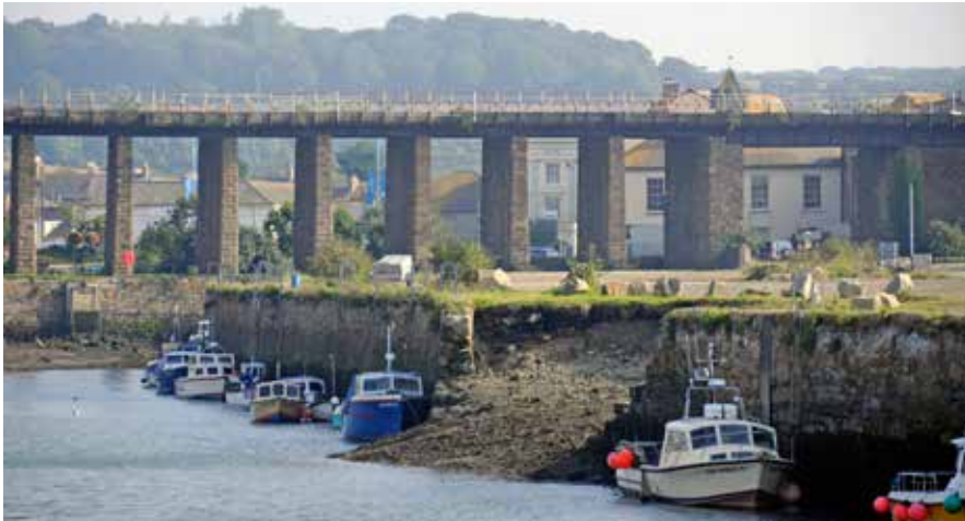
South Quay, Hayle, before conservation and construction of the store; note the significant breach in the quay wall here
