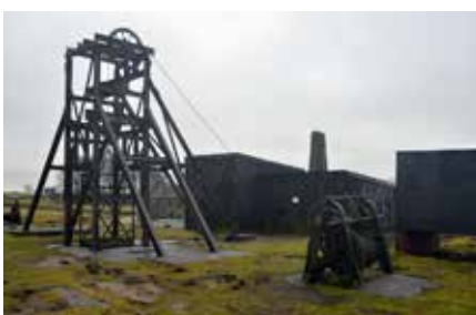
: The later steel winding headframe at Magpie (above left) with a reconstructed timber horse 'gin' (centre), and (right) the house of the original steam powered winder with surviving drum
