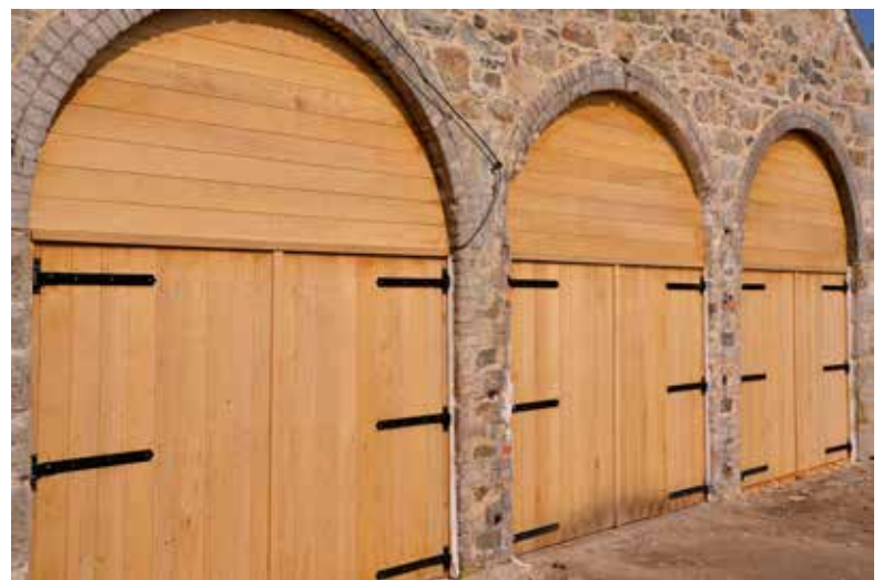
The boiler house doors, skilfully reconstructed by craftsmen of the Tregothnan Estate
