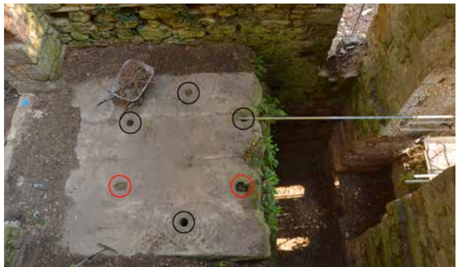
Vertical view of the engine cylinder bedstones showing where the mounting bolt holes have been cut or reshaped (within the red circles), presumably to accommodate the smaller diameter steam cylinder of c.1909
