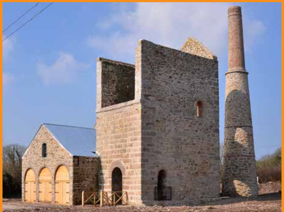
The engine and boiler houses with chimney at Wheal Busy, Chacewater, during and after conservation
