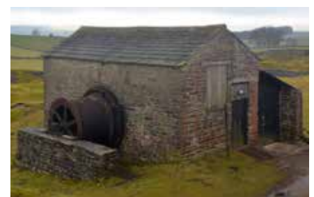
: The later steel winding headframe at Magpie (above left) with a reconstructed timber horse 'gin' (centre), and (right) the house of the original steam powered winder with surviving drum
