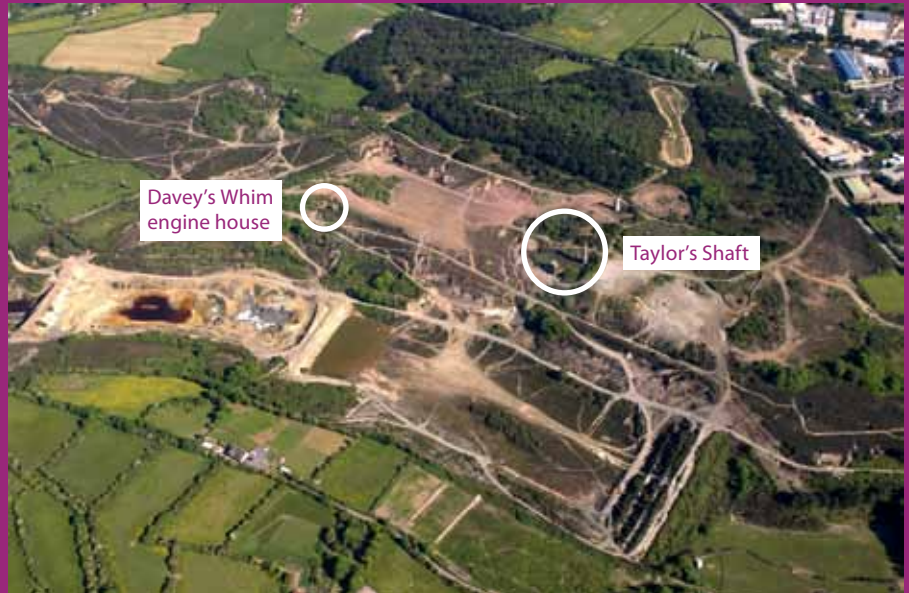
Aerial view of the Wheal Maid Valley, near Crofthandy, with the Consolidated Mines HLS project areas circled
