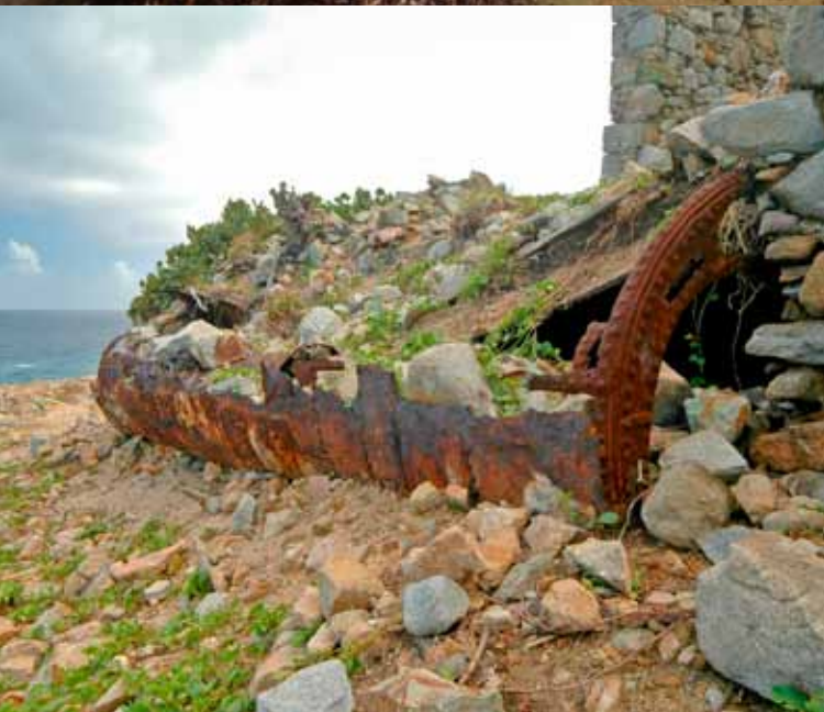
Top left: the cast iron side plates of the pumping engine beam, made at Perran Foundry, Perranarworthal, in the surf at Handsome Bay (© Lin Briggs); bottom left: a partially surviving Cornish boiler (© Simon Chapman)
