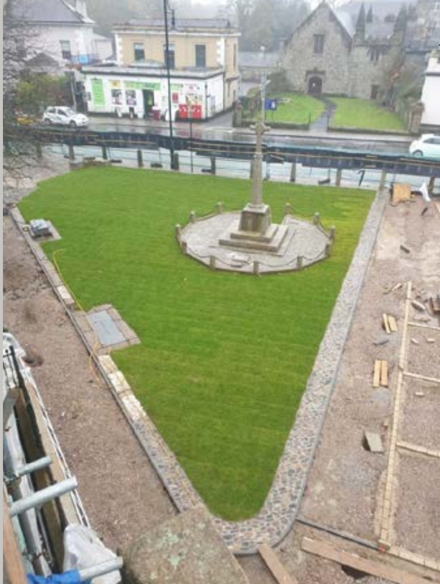
Right: The newly-redeveloped frontage to the Guildhall nearing completion
