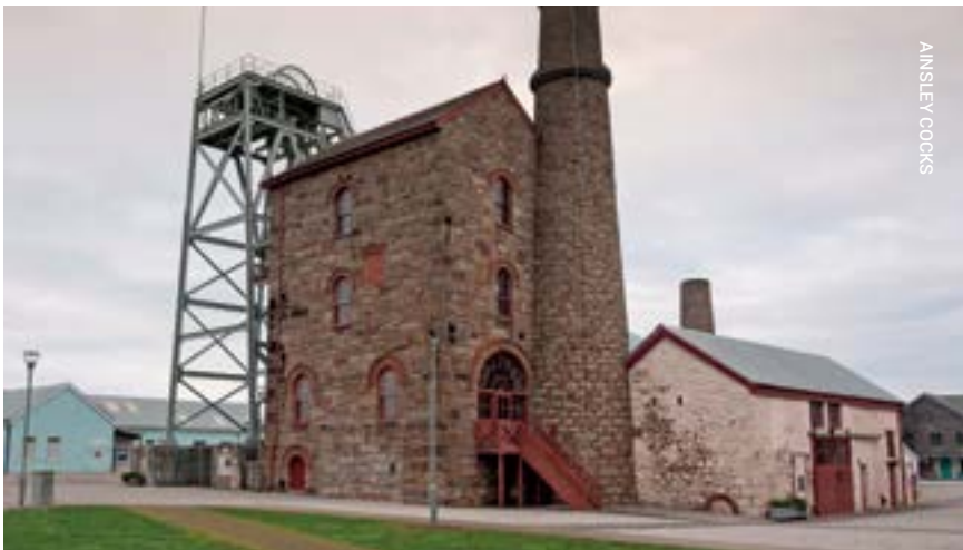
Above: Robinson's Shaft (Listed Grade II*). Above right: Botallack (Listed Grade II)
