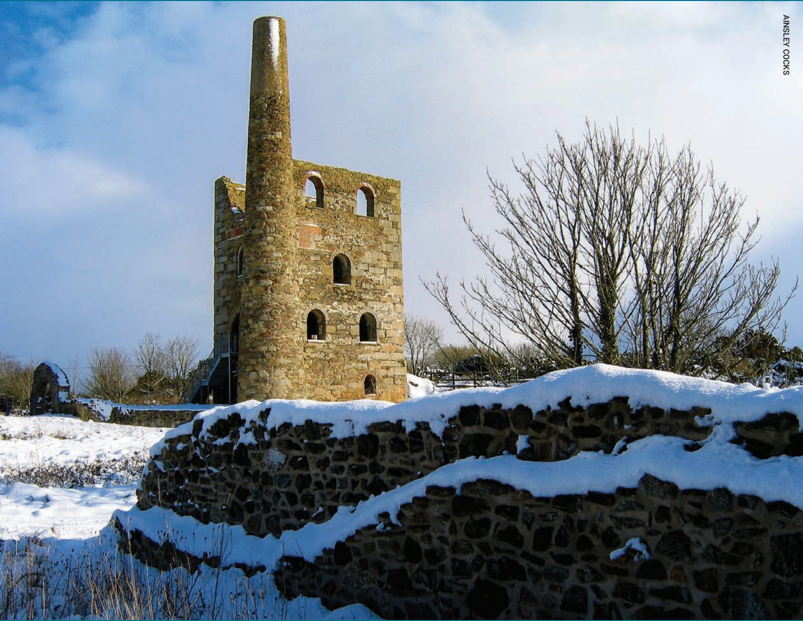
The pumping engine house at Wheal Peevor, near Radnor, February 2009
