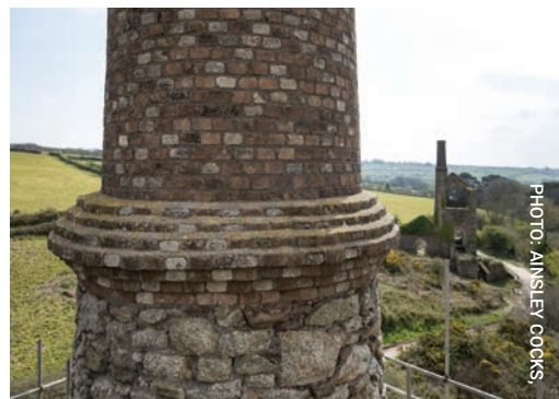
Above: Stack repairs at the Pascoe's Shaft Pumping Engine House
