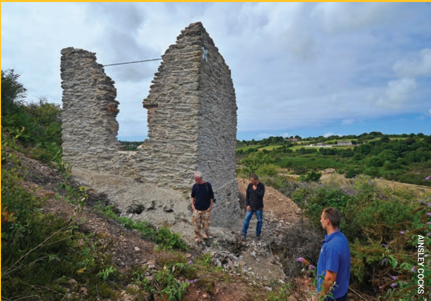
Top: The Taylor's Shaft Pumping Engine House and boiler chimney following conservation
