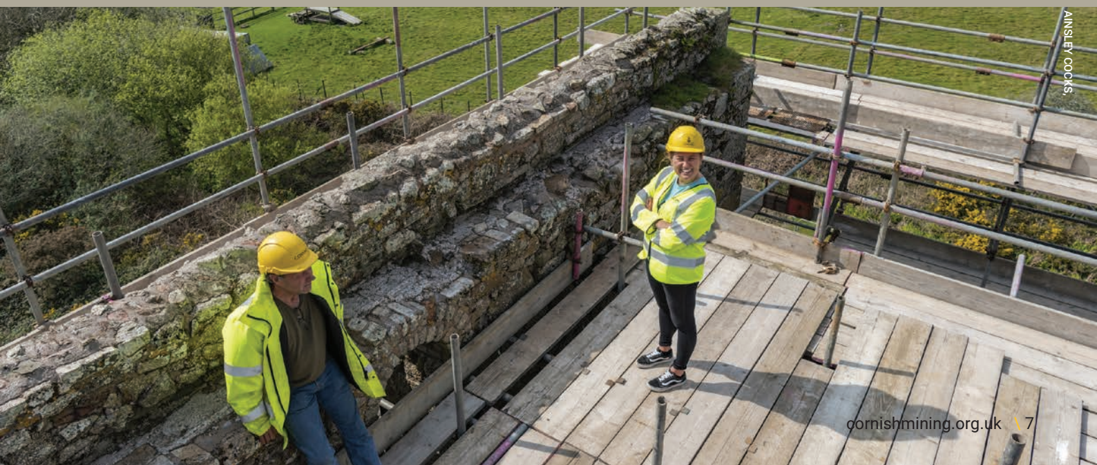
Above: The engine house cylinder arch opening, sized to accommodate the diameter of the engine steam cylinder
