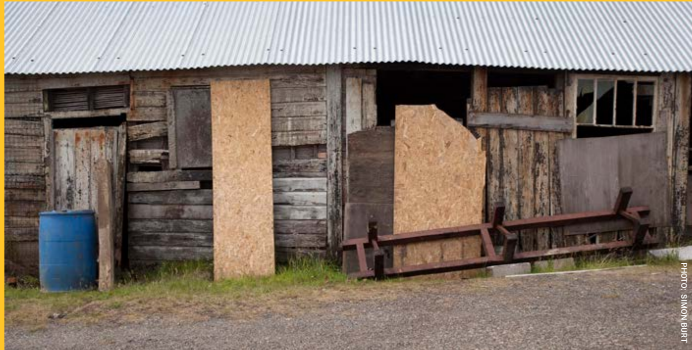
Below: The mine Assay House prior to conservation works (2014)
