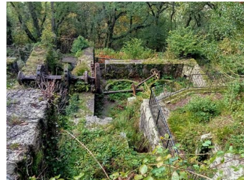
Below: Carmears wheel pit before clearance Bottom: Carmears wheel pit after clearance
