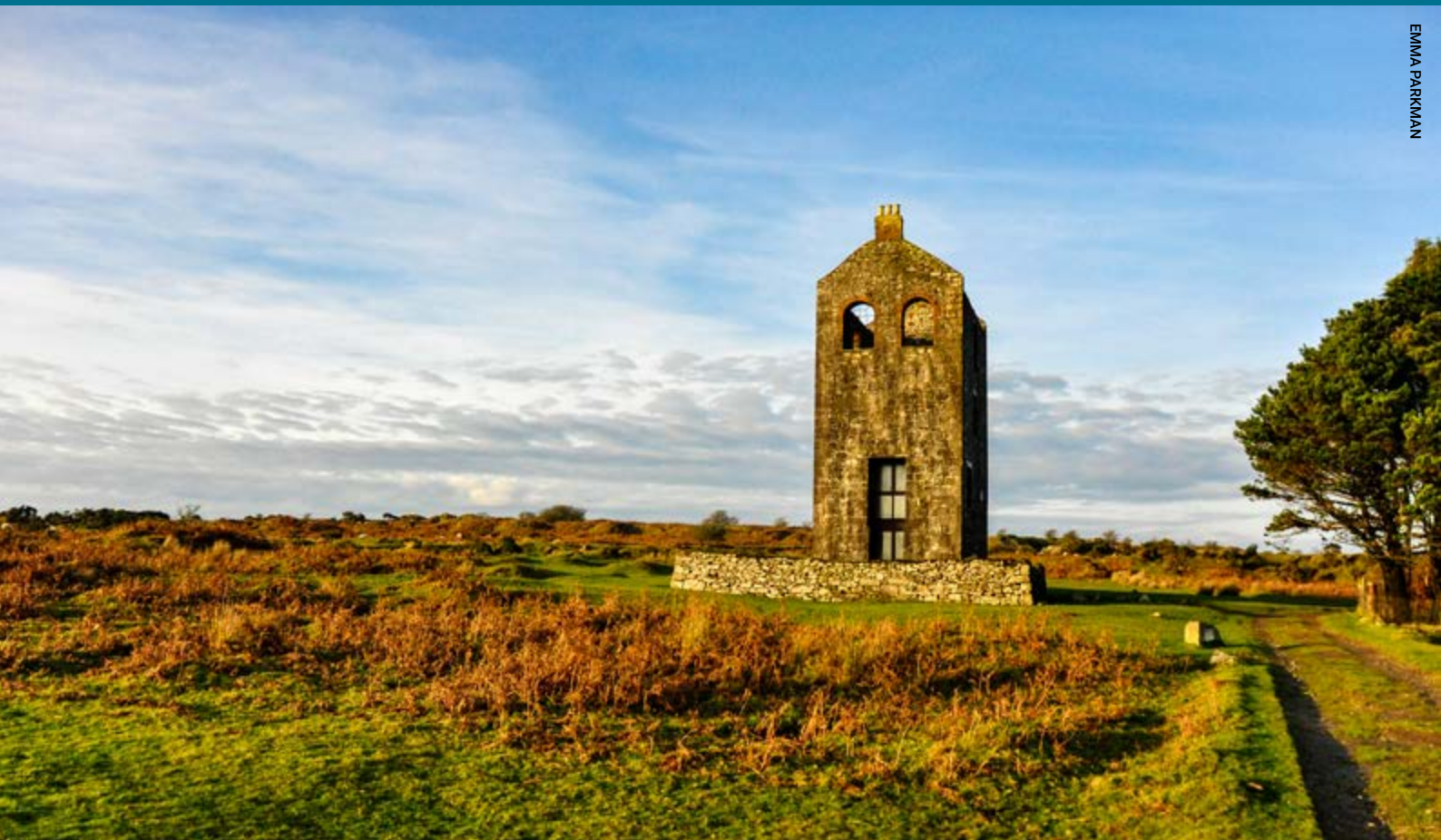
Houseman's Shaft Engine House, South Phoenix Mine, November 2020
