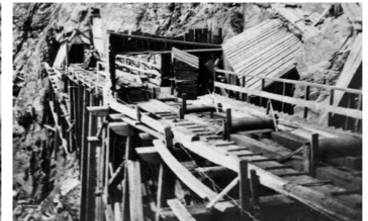
An alternate view showing a waggon with mineworkers just outside of the Boscawen Diagonal Shaft portal (upper left), c.1865-1866. (Charles Renowden Lobb - The Stephen Colwill Collection)
